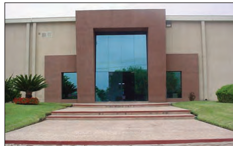
Monterrey, Mexico Manufacturing and Distribution
