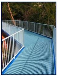
Pultruded fiberglass grating is uni-directional in strength and provides increased load capacity and very good levels of corrosion resistance. The components (bearing bars and cross bars) which are pulled by machine, provide a higher glass to resin ratio content (65% glass to 35% resin) which gives it superior load capacity, yet reduces the corrosion resistance when compared to molded fiberglass grating.
