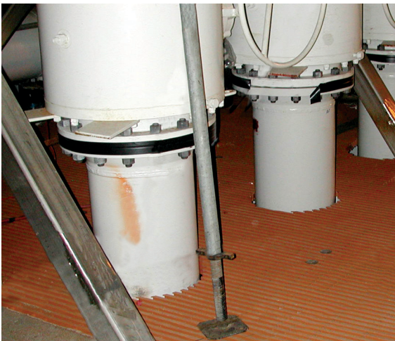
DURAGRID® Phenolic Grating's unique construction allows for many penetrations to be cut without adding additional supports.
